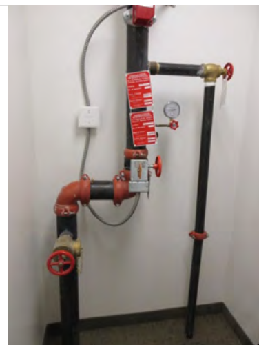
84. Fire riser in stairwell
