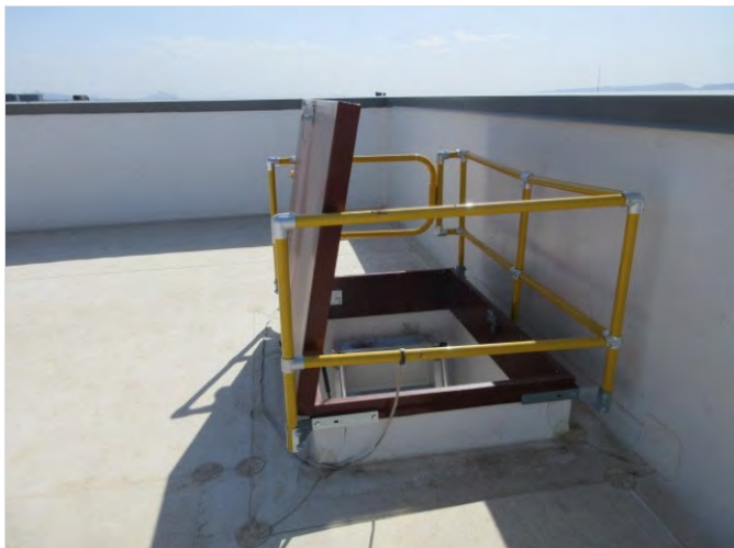
85. Roof access hatch
