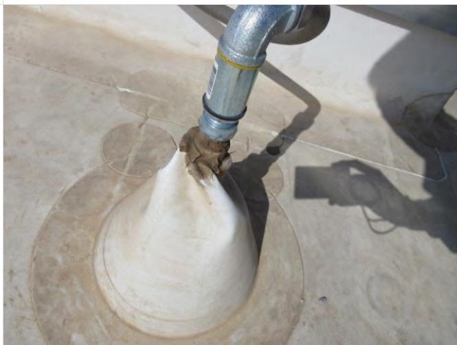
88. Collapsed roof penetration boot
