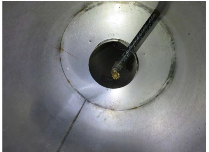
82. Fire sprinkler in linen chute
