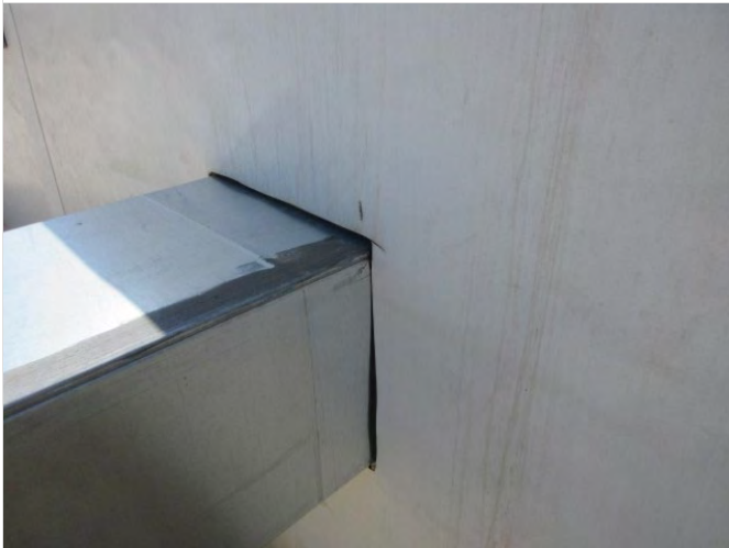
93. Missing flashing
