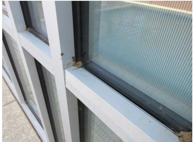
100. Excessive caulking at storefront windows adjacent to pool
