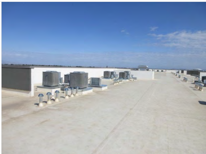
86. TPO roof membrane
