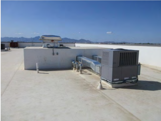
91. Elevator shaft package unit
