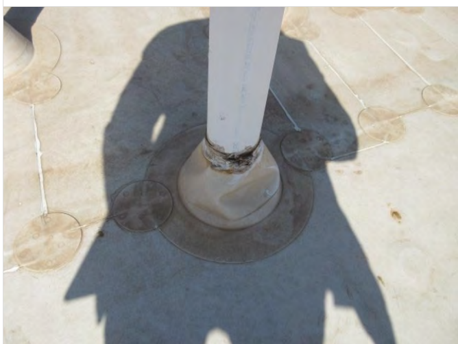
89. Collapsed roof penetration boot
