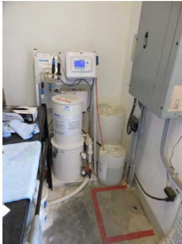
45. Pool chemical feed equipment
