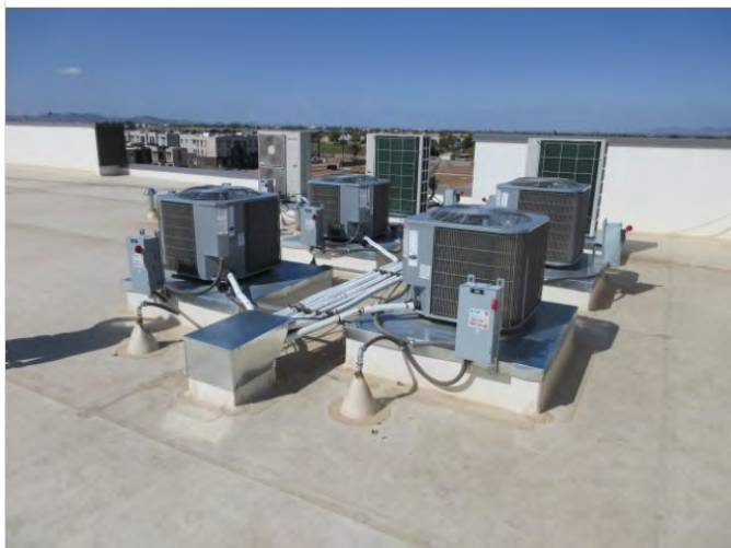
87. Rooftop mounted HVAC equipment
