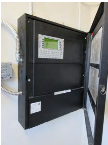
47. Fire alarm control panel
