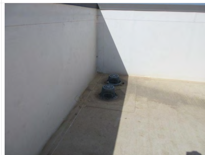
90. Roof drains (primary and secondary)
