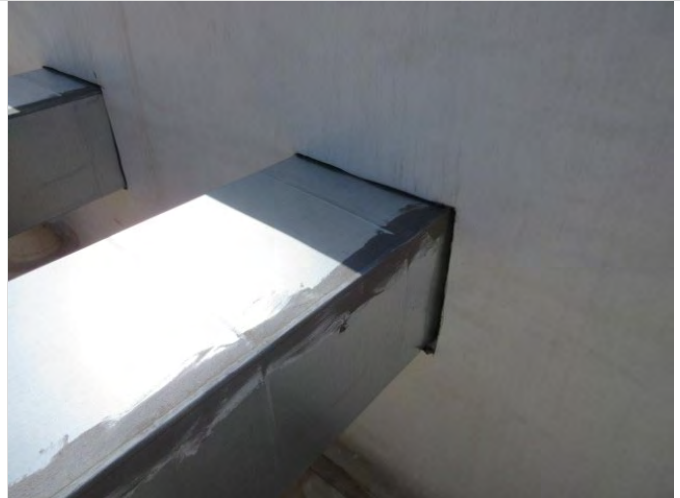
92. Ducting from package unit to elevator shaft, missing flashing
