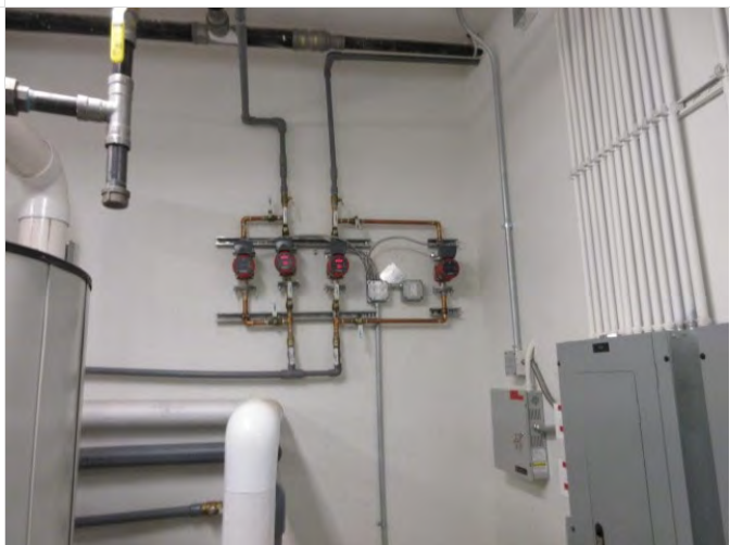
30. Hot water recirculation pumps
