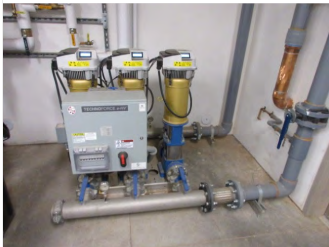
29. Domestic water triplex pump system
