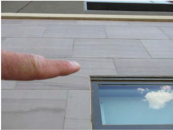
51. Cracked exterior tile
