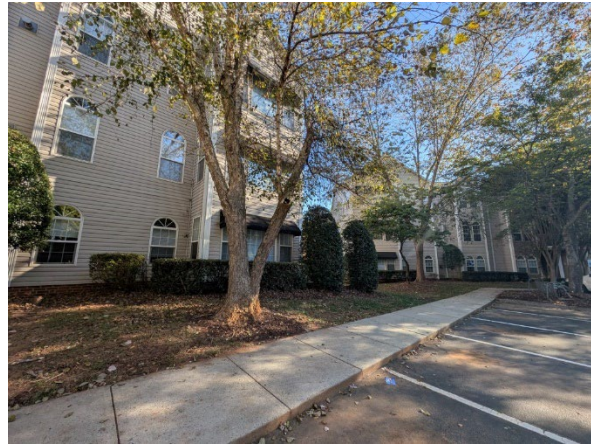
View of Subject Exterior
