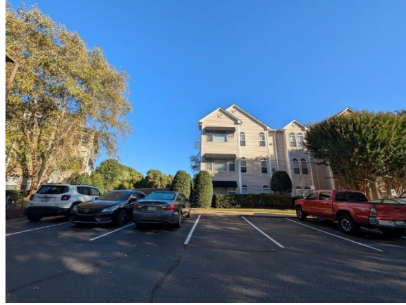
View of Subject Exterior
