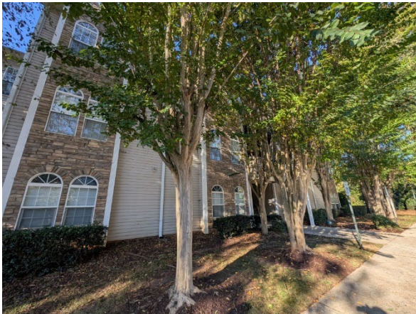
View of Subject Exterior
