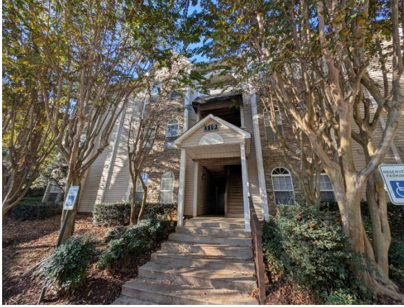
View of Subject Exterior
