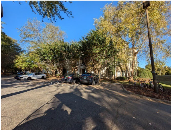
View of Subject Exterior
